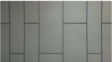
Offset joint vertical installation
