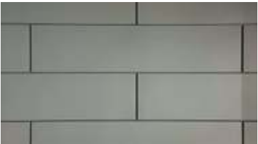
Offset joint horizontal installation
